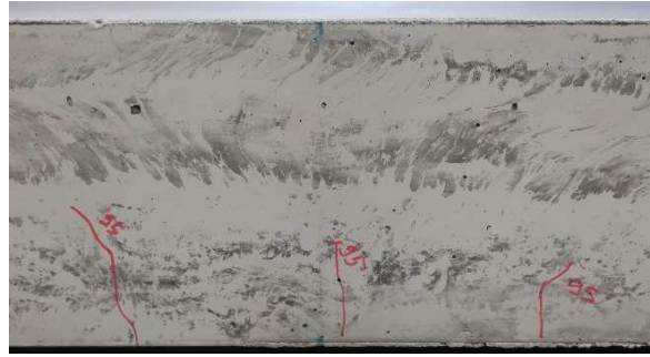
Figure 11. Test C1A: Vertical cracks at the middle span of the slab.
