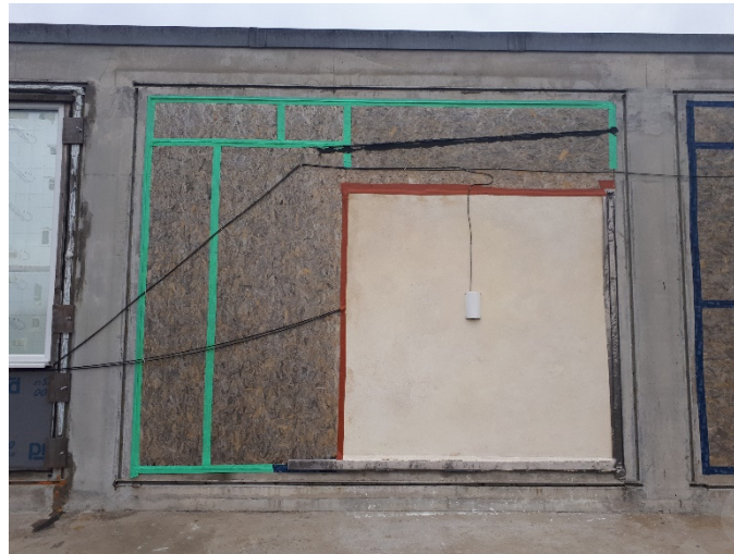
Figure 7: Outer face of the instrumented ISOBIO wall – HIVE demonstrator (Wroughton, UK)
