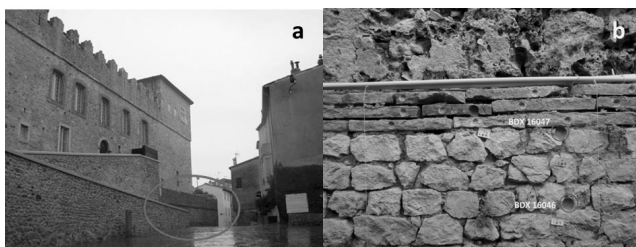
Figure 2: (See colour plate II) a) View on the west face of the castle, the gallo-roman foundations marked in a red circle; b) Wall MR 10003 after sampling of both bricks and mortars, before restoration.
