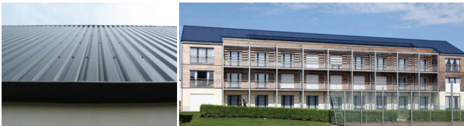
Fig.1 - a) SolarWall Collector ; b) Maisel site using solar collectors
